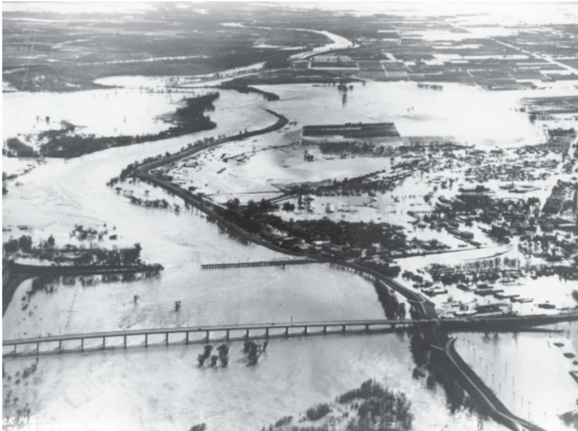
Figure 1: Photograph of 1955 Levee Break with 10 th Street Bridge in the Foreground (Source: Sutter Butte Flood Control Agency Special Publication, Flood Aware/Flood Prepare)
